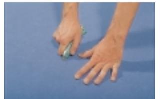
A useful tip if the trapped air cannot be forced out laterally: make a small hole with the point of a blade in a dark section of the pattern, press out the air and once again firmly rub down the covering at this point.
