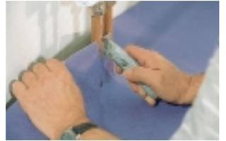
The loosely-laid sheets are cut in, around a radiator in this case.
