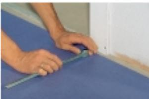
Transferring the shape of a doorpost to the linoleum with the help of a bevel.
