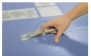
The weld rod is trimmed in two operations, first with the trimming guide fitted, then with the bare blade.
